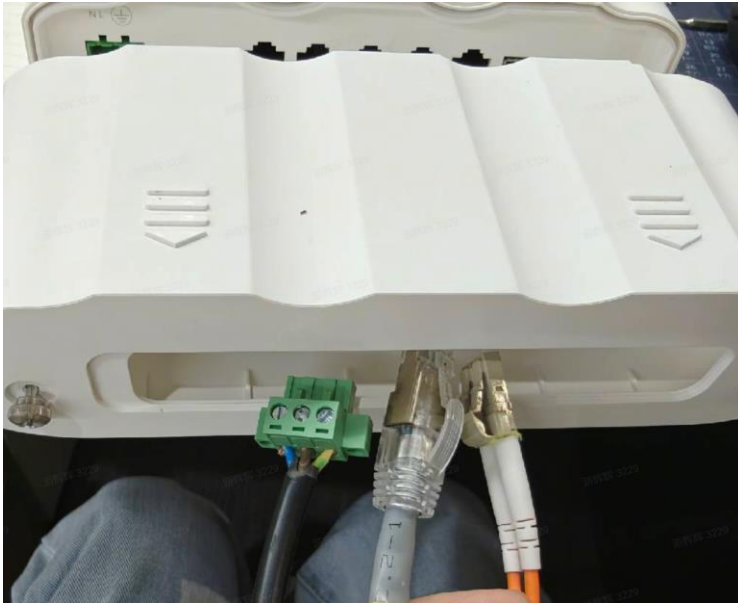
Figure3-7 Connecting Cables to the Equipment (4)
