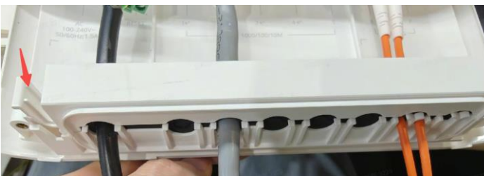
Figure3-11 Connecting Cables to the Equipment (8)
