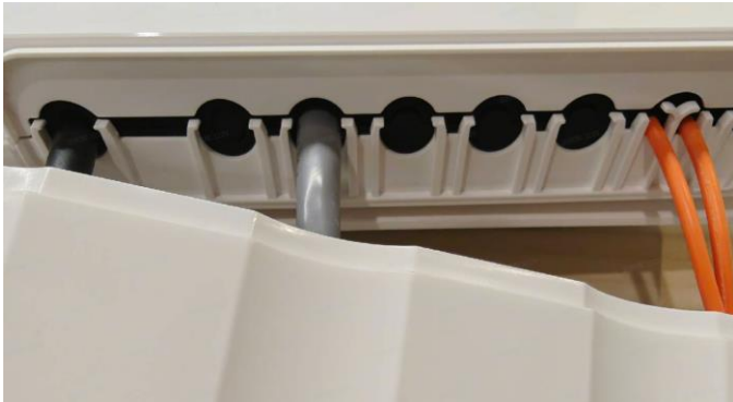
Figure3-12 Connecting Cables to the Equipment (8)
